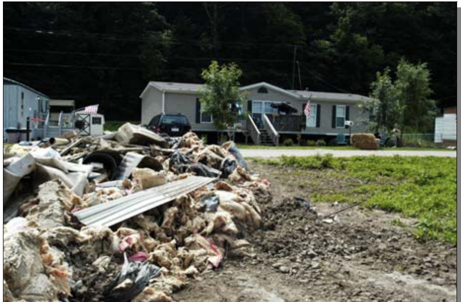
Quinland, WV, June 30, 2003 -- This home, elevated above the Base Flood Elevation, received no damage during the recent flooding here. The flooding devastated much of the rest of the homes in the neighborhood. Photo by Liz Roll/FEMA News Photo
