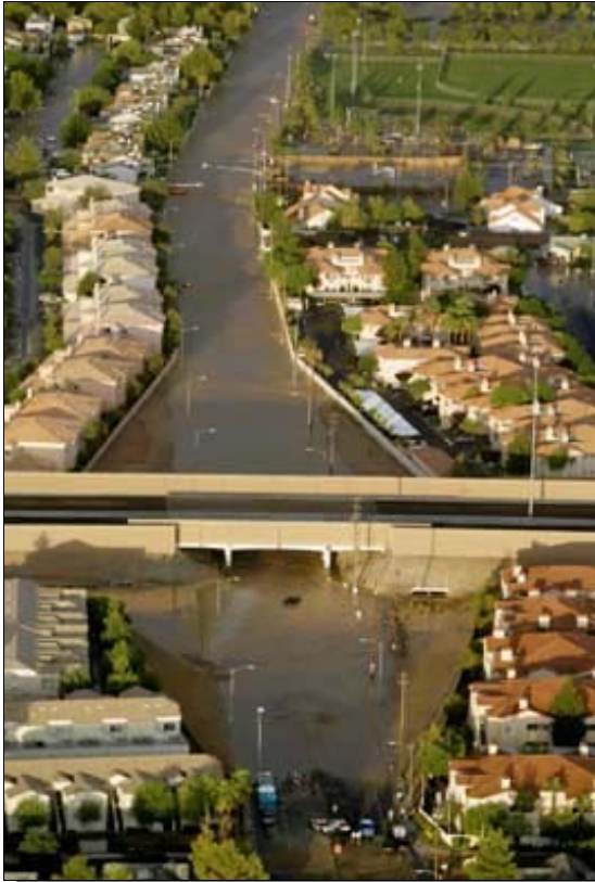
Floodwaters submerge Gowan Road under U.S. Highway 95. Photo by K.M. Cannon, courtesy of the Las Vegas Review Journal.
